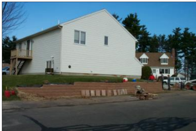
Country Hill Rd. and McTavish Dr. after replacing timber walls.
